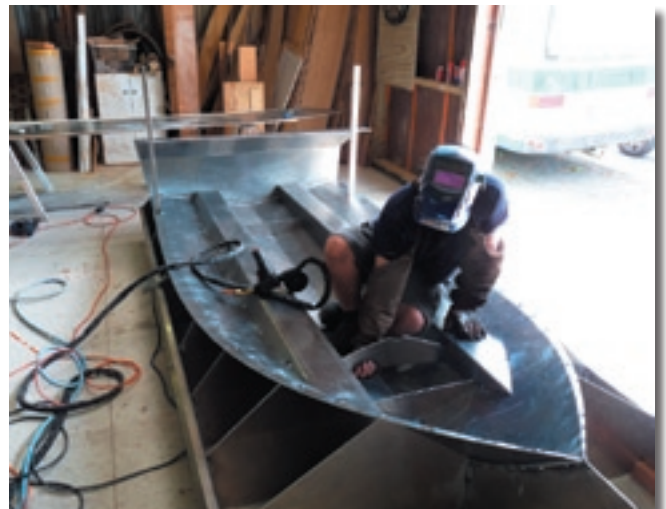
Spacers and tack-welded girders in place.
