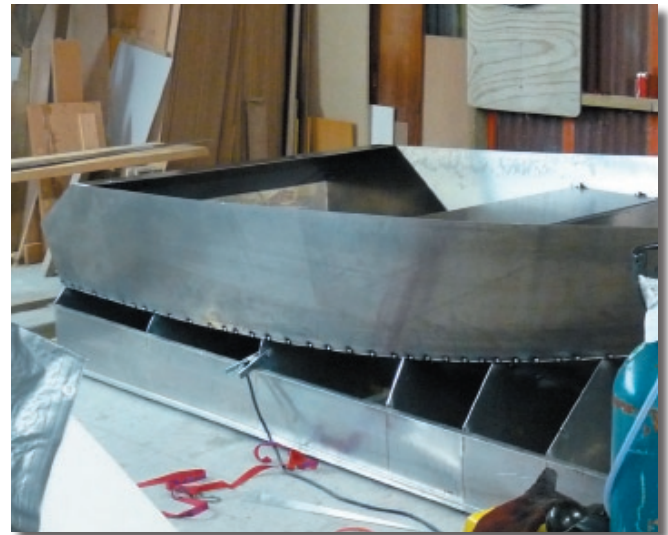
Tack-welded seams will be fully welded on both sides.
