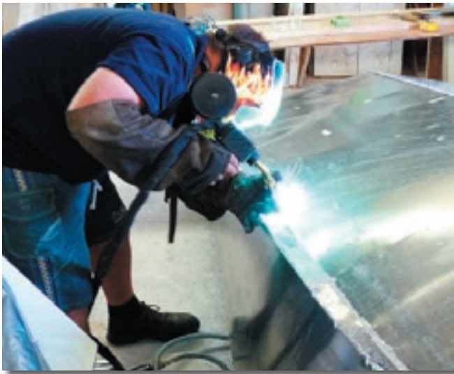
Finishing outside welds.
