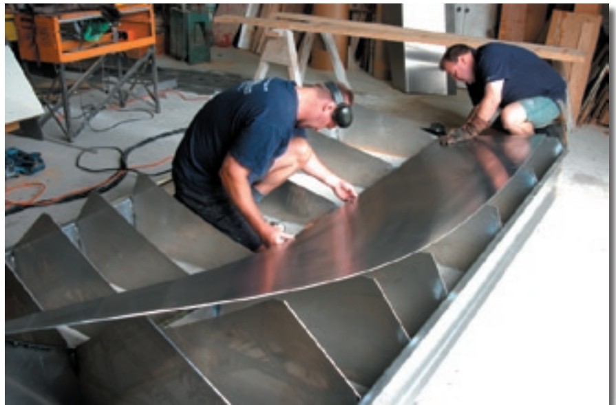
Jim and Jason fit bottom panel into aluminium jig.
