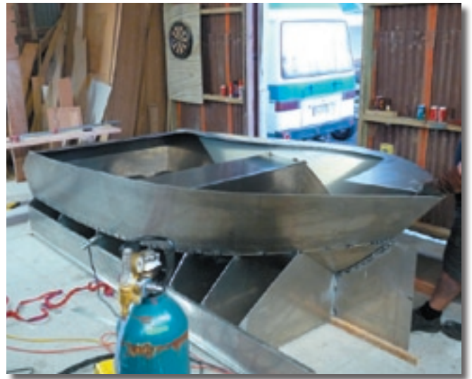
Deck panels set up.
